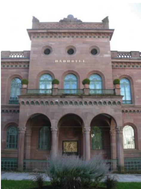
Palais Thermal (Eberhardsbad) in Bad Wildbad
