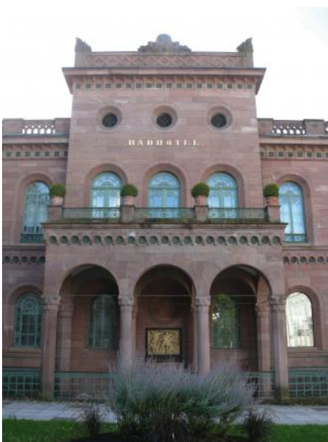
Palais Thermal (Eberhardsbad) in Bad Wildbad
